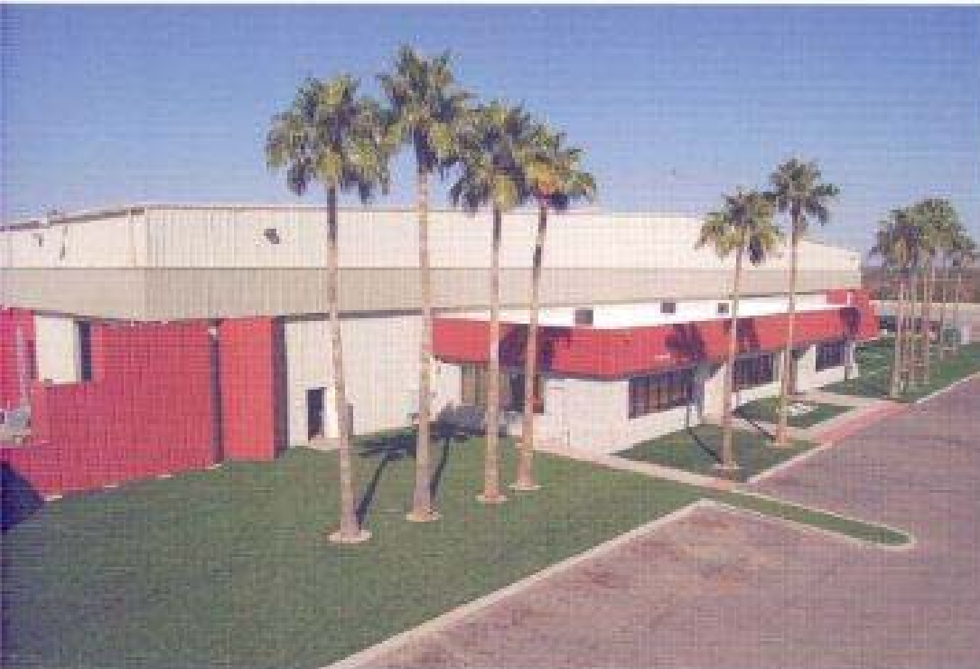
The Arizona CRM plant, a major supplier of crumb rubber for synthetic turf, installed 28,000 square feet of the material around its building and parking lot. The project used 8400 tires and eliminates landscape maintenance and watering costs as well as cutting the desert dust. Photo by Terry Eitel
