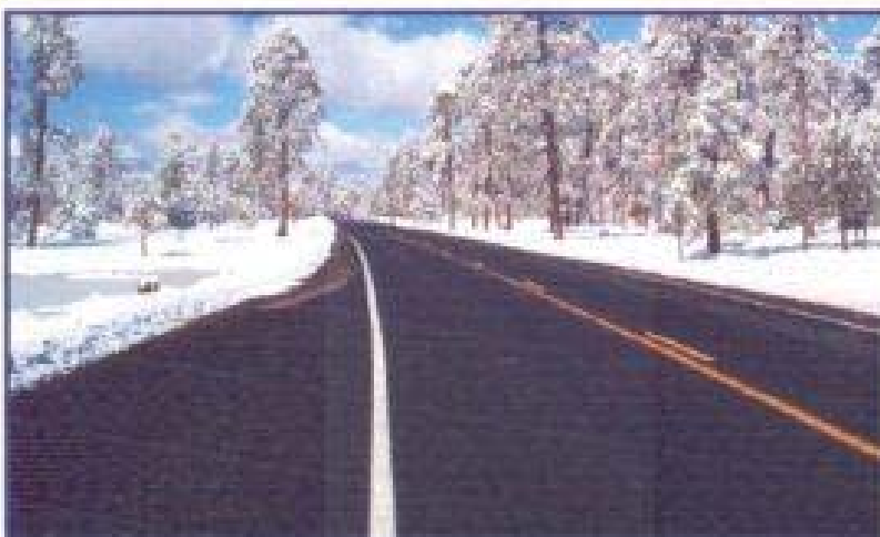
Asphalt Rubber Pavement on State Highway 260 in the Arizona high country. Typical rubberized pavements contain 20% crumb rubber and 80% asphalt. The rubber modified asphalt provides a smoother, quieter ride, retards aging and cracking, better skid resistance and longer service life.
